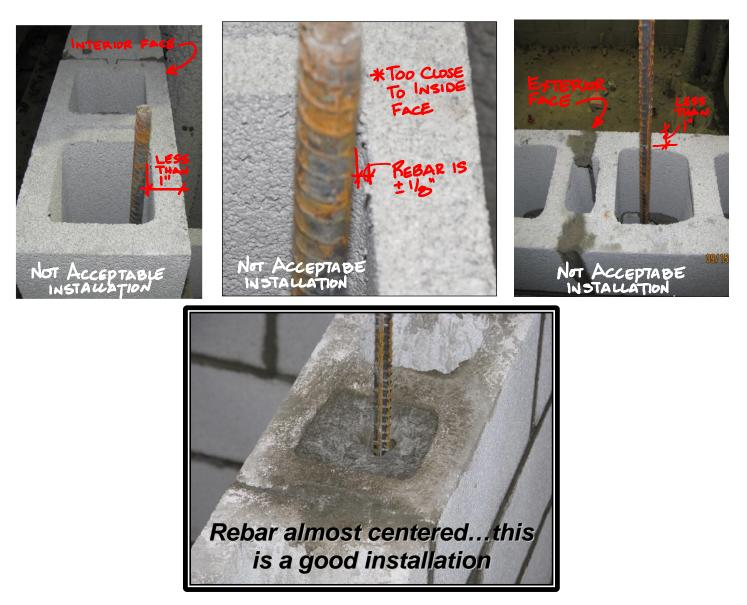
When THE CMU is exposed to the weather, the edge of the rebar must be no closer than 2" (for a #6 or greater) or  $1 \frac{1}{2}$ " (for a #5 or less) from the face of the exterior portion of the CMU.
